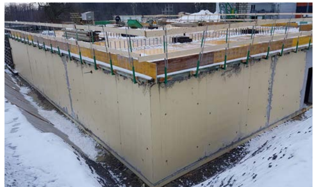
Open excavation with SikaProof® A+: After removing the formwork, the anchor penetrations have to be sealed.
