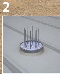
SikaProof® detailing solutions, e.g. for pile caps
